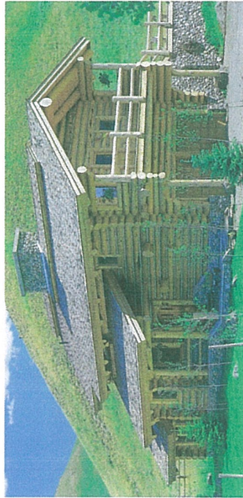
▲ Deck overhang & large log columns de-emphasize the garage doors below.
